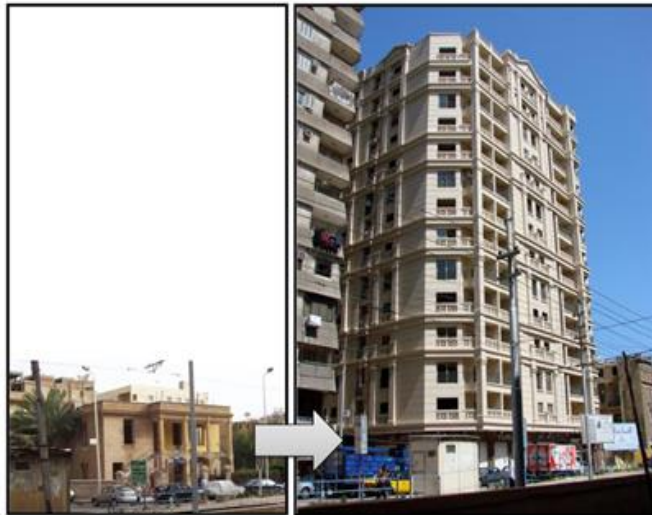
Fig. 1. A small villa in El-Raml area demolished to make way for a huge apartment building. Source: internet picture
