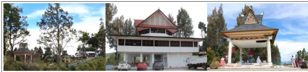
Fig. 2: Existing Buildings in Sipiso-Piso waterfall
