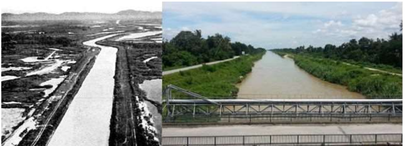
Figure 2: The canalization of Kinta River involving 61km length, from Ipoh to Kuala Chenderiang. Source: Old photo reproduced from (Khoo & Lubis, 2005, p. 325); new photo was photograph by author in 2018.
