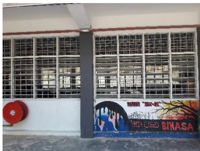
Figure 7. The classroom in CD
