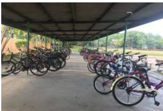
Fig. 3: The shaded and safe bike parking inside the school.
