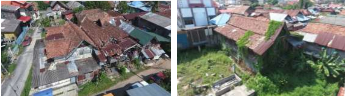
Fig. 2: The demise of traditional Malay architecture (Source: Abdullah, 2021)
