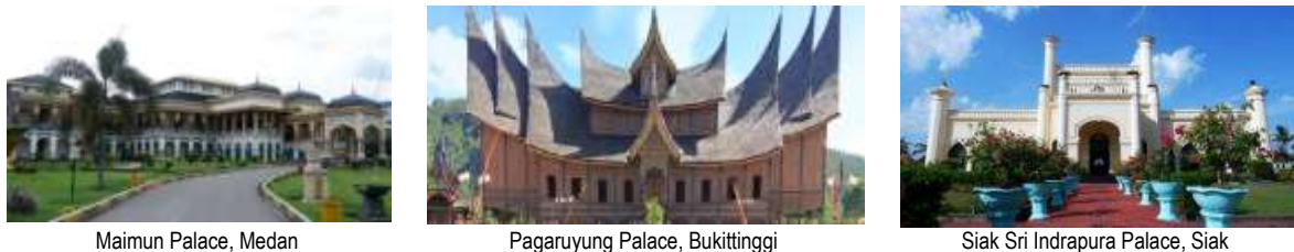
Maimun Palace, Medan Pagaruyung Palace, Bukittinggi Siak Sri Indrapura Palace, Siak Fig. 2. Cultural Building of Heritage Tourism (Source: Author)
