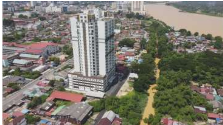
Fig. 12: View of S.K Condominium (Source: Azli Abdullah, 2019)
