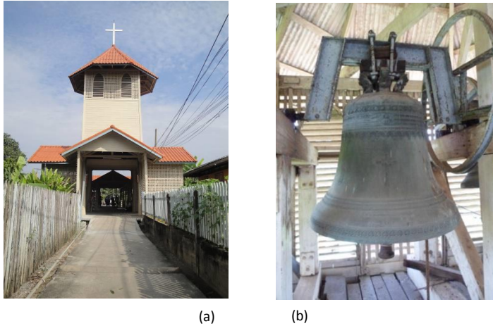
Fig. 5. (a) The Bell Tower and the Rest Pavilion; (b) The Bell
