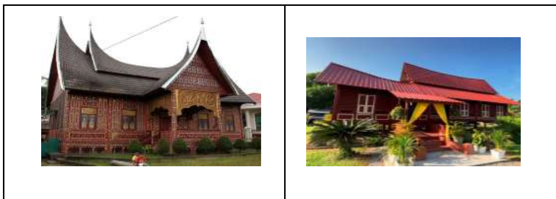
Fig. 11: The roof shape difference between Minangkabau (left) and RTAIS (right) can be seen through the " lentik "- the RTAIS ridge line is built with slight upward curves without the outward protrusion. (Source: Author, 2022)
