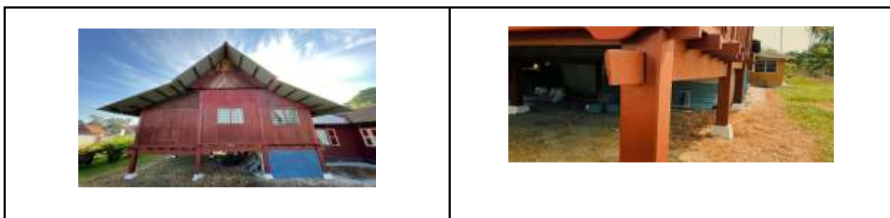
Fig. 14: A raised floor on stilts protects against flooding and animals. (Source: Author, 2022)
