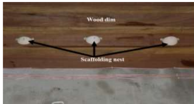
Fig. 11: Installed scaffolding nest in swiftlet's house
