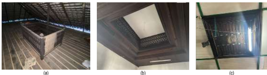
Figure 5: Variation of peeping gallery and screen (a) the peeping gallery of House No. 1 viewed from the padong . (b) the peeping gallery of House No. 2, viewed from tengah , now has been sealed. (c) the peeping screen of House No. 3 viewed from tengah . (Source: Researcher's fieldwork)
