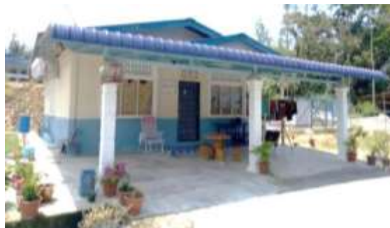
Fig. 6: New porch constructed in RKB2 (Source: Author)
