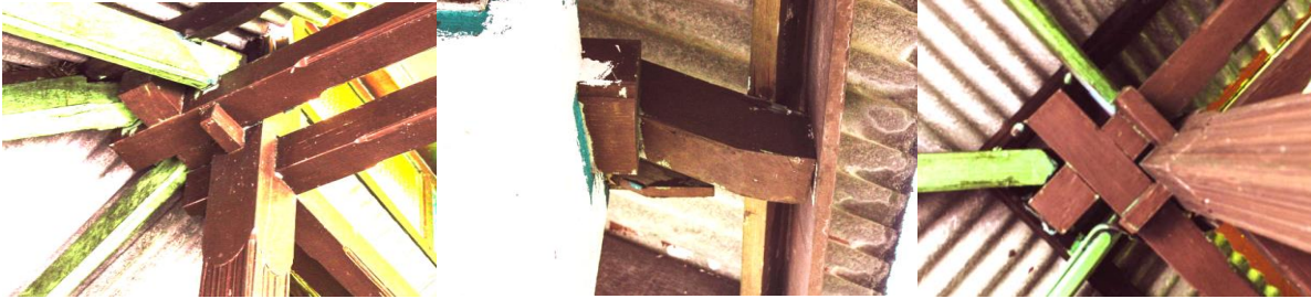
Fig. 3: Traditional tanggam construction on the roof of Masjid Jamek Tanah Datar (Source: Author, 2023)
