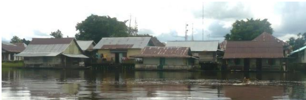
Fig. 3. Floating houses in Kampung Tumok. On the back are stilt-houses that are connected to each other using wooden pathways
