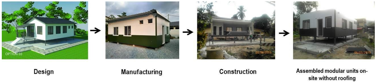
Fig. 5: The design, manufacturing and construction stages for case study B
