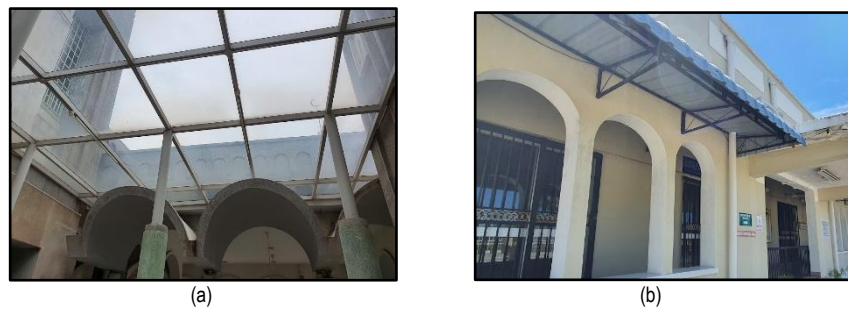
Fig. 6. Additional roof structure
