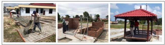
Fig. 6: Implementation works (Hardscapes) Hardscape works involves construction of planter box, pedestrian walkway, pump house and gazebo. (Source: Author (2018))
